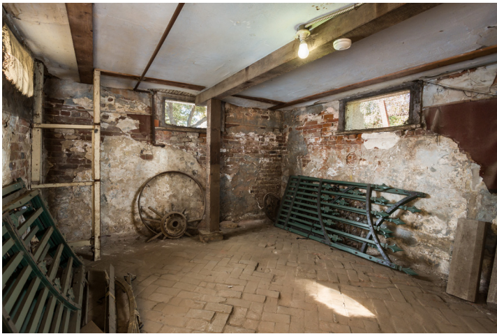
The basement of the Workman House.
