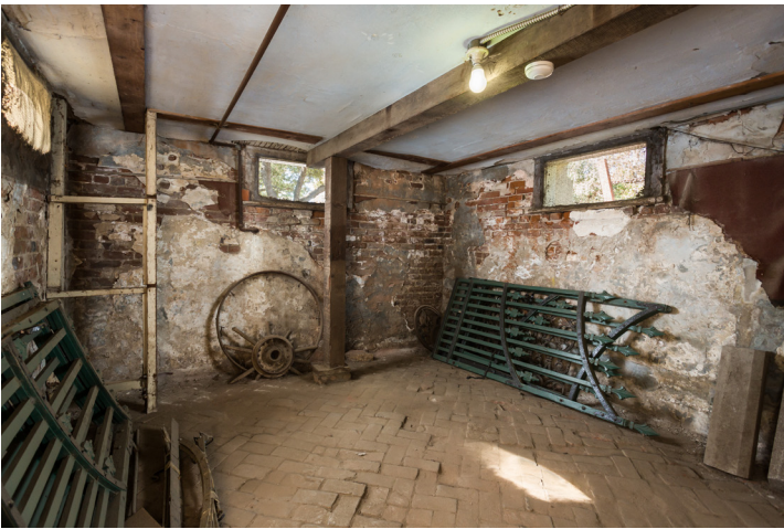
The basement of the Workman House.
