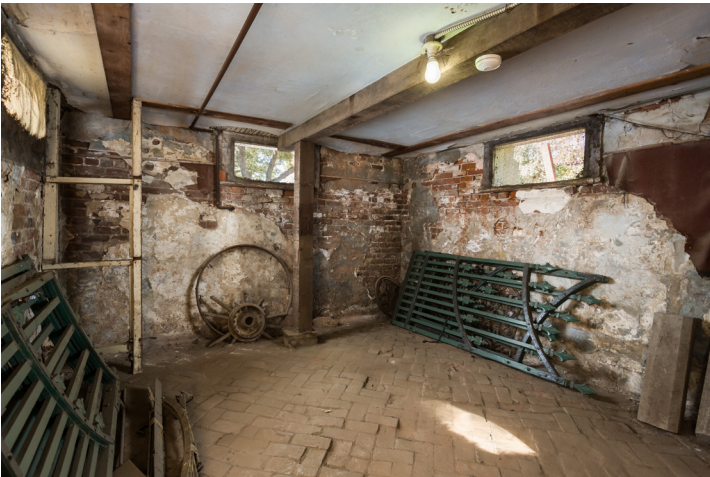
The basement of the Workman House.
